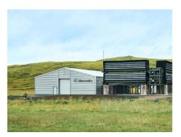
Climeworks Direct Air Capture technology uses only renewable energy and the modular CO<sub>2</sub> collectors can be combined to create machines of any size.
